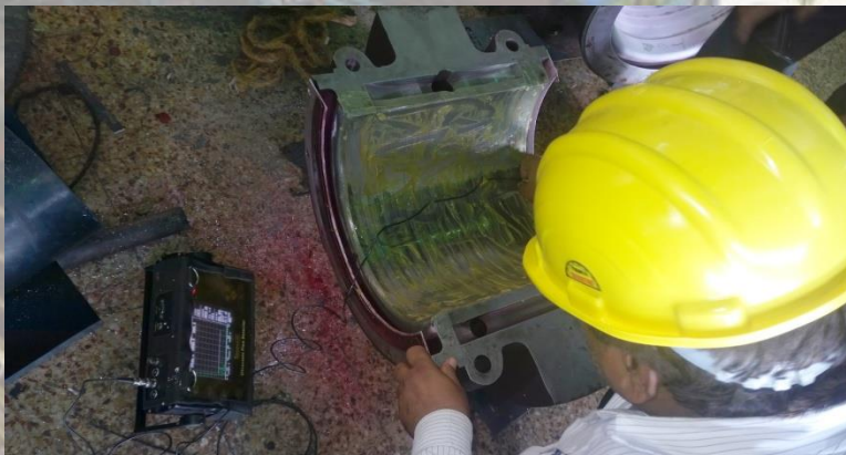
Ultrasonic Testing of Bearing being carried out
